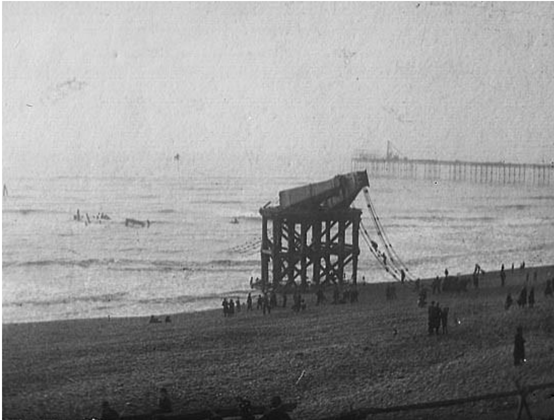
Wreckage of Chain Pier after Great Storm, 5th December 1896
